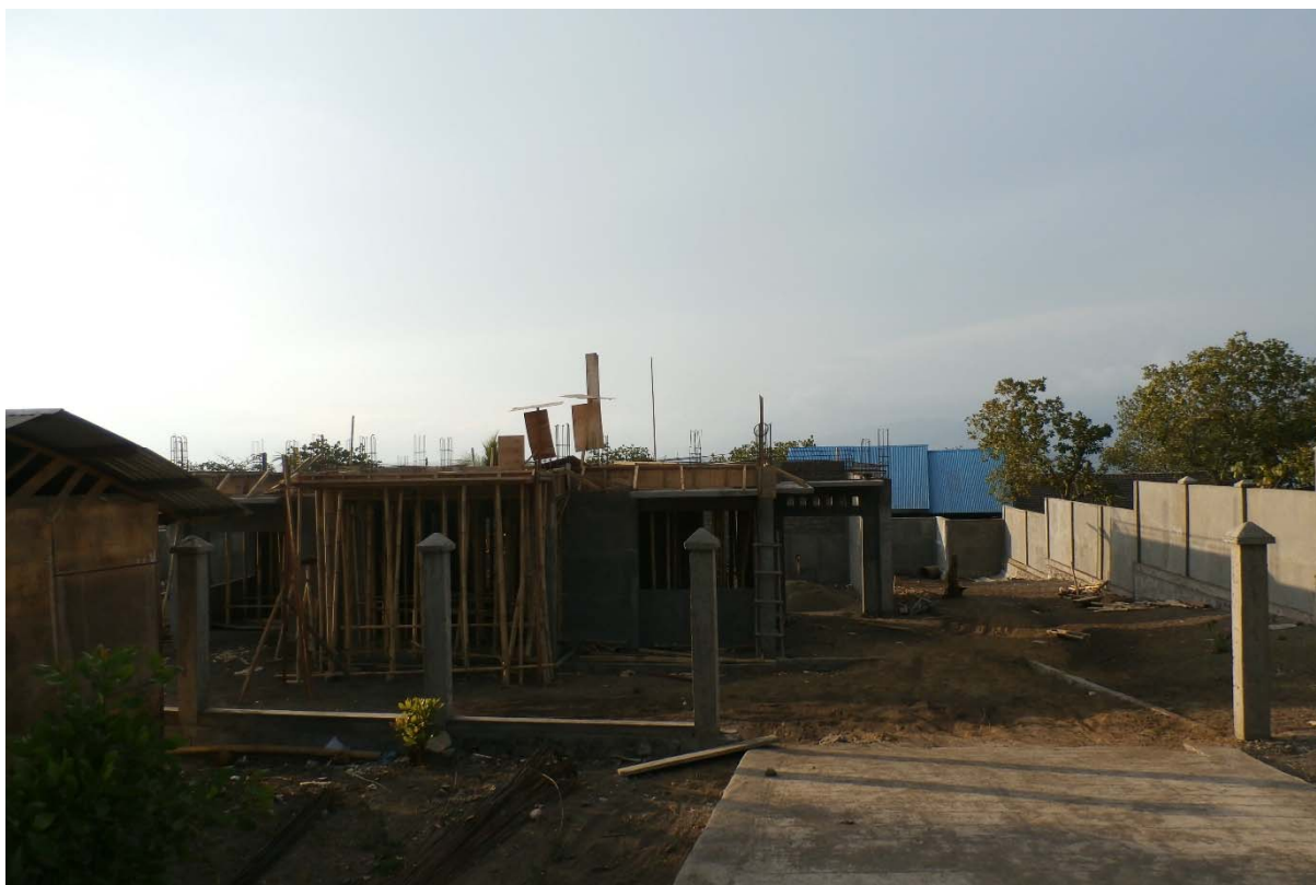
The construction of the Sea Water Reverse Osmosis (SWRO) at Pulau Ende.
